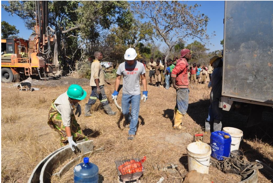
Students assisting drillers in installing the casing.
